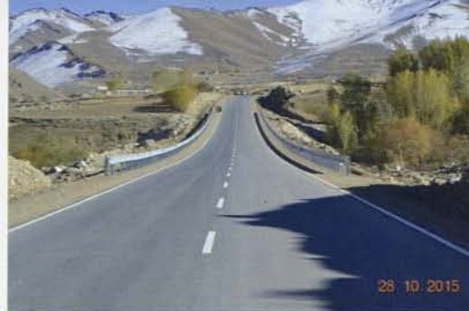
Bamyan-Onay Road , Afghanistan Type : National Highway Length : 142 km, Lane : 4-lane
