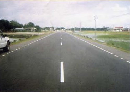
Dhaka-Khulna Road , Bangladesh Type : National Highway N8 Length : 163 km, Lane : 2-lane Connection : Mongla Port & southern districts
