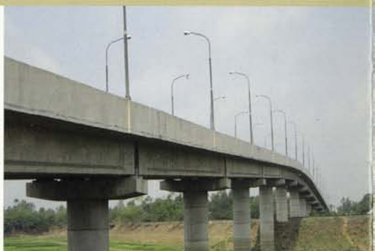
Kaliakoir Rail Bridge, Bangladesh Type : Pre-Stressed Concrete Dimension : Length 435 m, Width : 20 m
