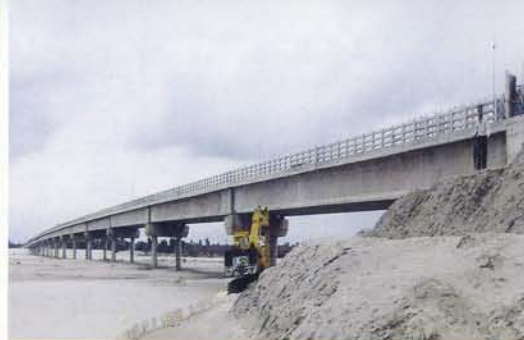
Teesta Bridge, Bangladesh Type : Pre-Stressed Concrete Dimension : Length 750 m, Width : 20 m
