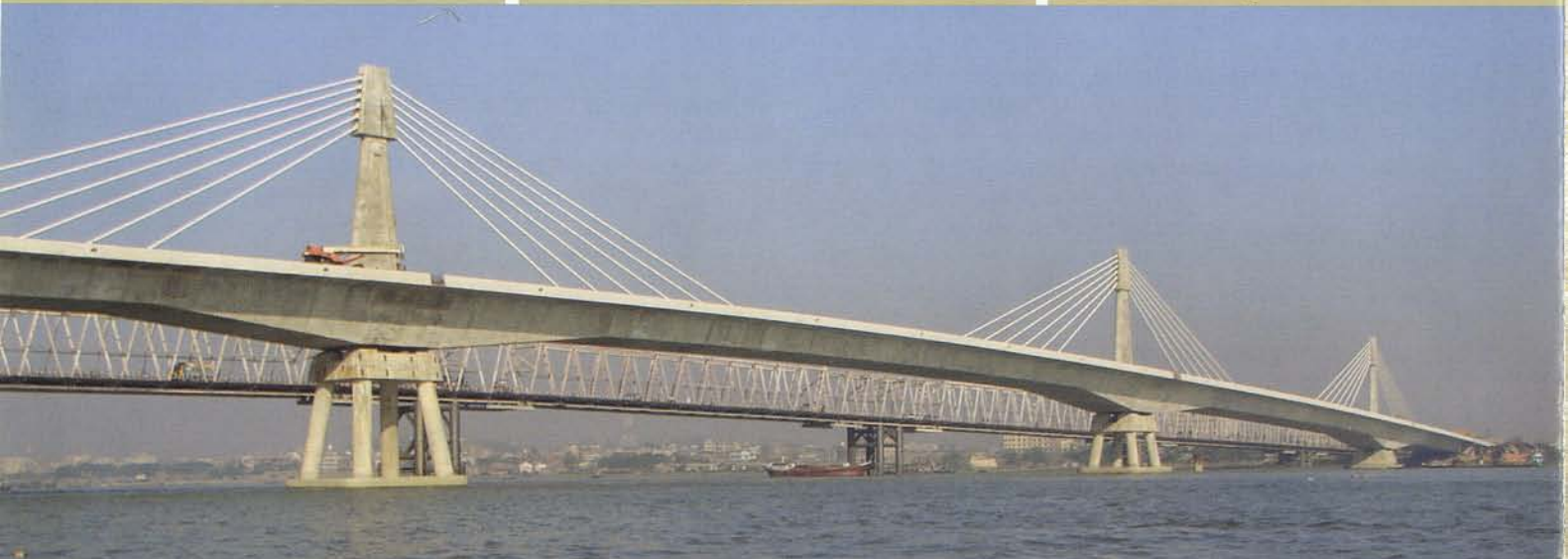
Shah Amanat Bridge, Bangladesh Type : Extradose PC Box Girder, Dimension : Length 950 m, Width : 24 m
