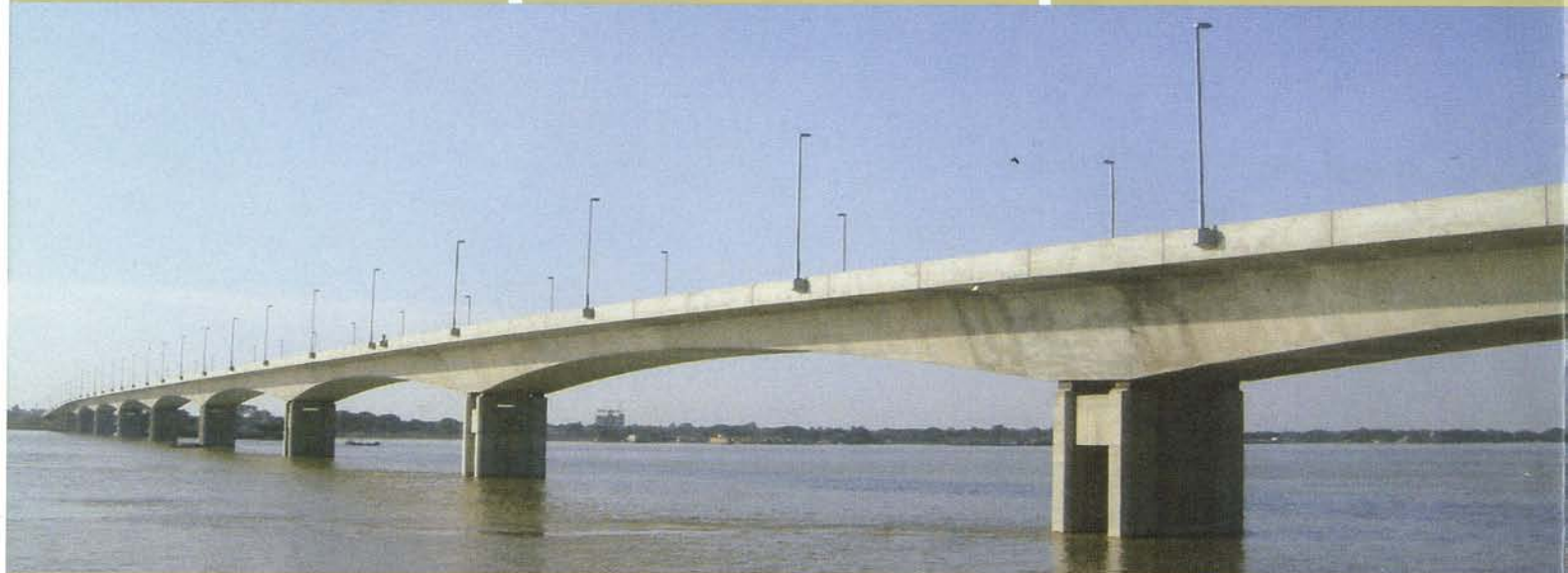
Bhairab Bridge, Bangladesh Type : Pre-Stressed Concrete, Dimension : Length 1023 m, Width : 24 m
