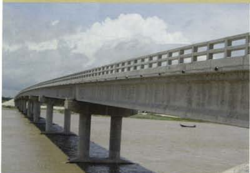
Shariatullah Bridge, Bangladesh Type : Pre-Stressed Concrete Dimension : Length 450 m, Width : 20 m
