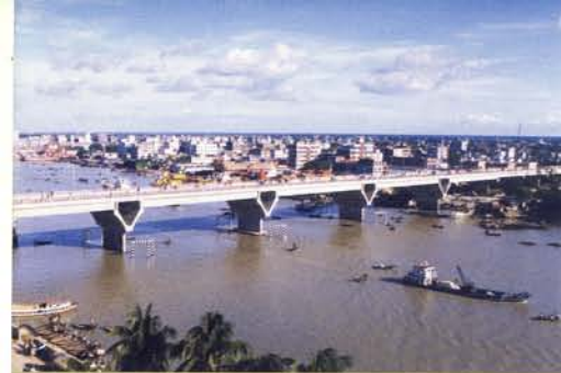
Muktijodhah Bridge, Bangladesh Type : Pre-Stressed Concrete Dimension : Length 1170 m, Width : 20 m
