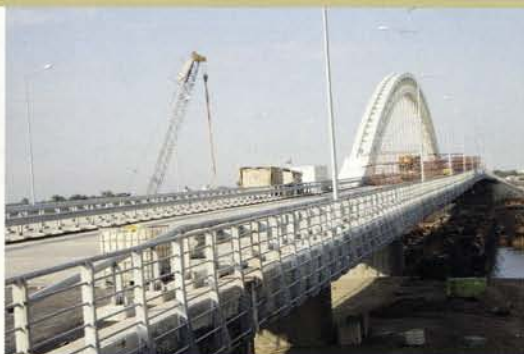
Salyan Bridge, Azerbaijan Type : Pre-Stressed Concrete Dimension : Length 360 m, Width : 20 m
