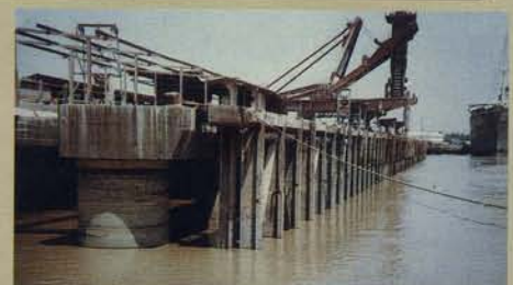
Cement Clinker Jetty, Bangladesh
