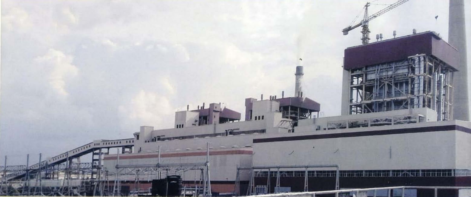
Barapukuria Coal Fired Thermal Power Station 275 MW Project, Bangladesh
