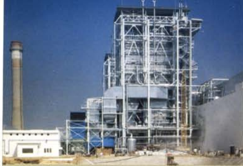
Raozan Power Plant, Chittagong, Bangladesh
