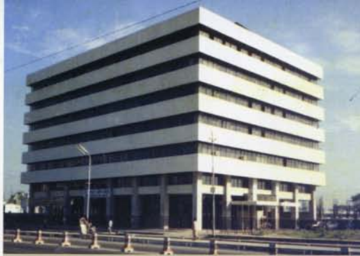
BSEC Building, Bangladesh
