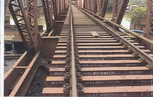
Dhaleswari Rail Bridge, Elenga, Bangladesh
