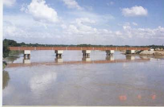
Pungli River Railway Bridge, Bangladesh
