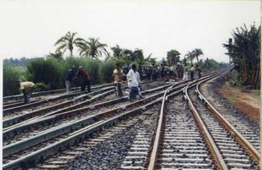
Fixing Track at Santahar JBRLP, Bangladesh
