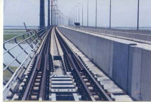
Bangabandhu Bridge Rail Track, Bangladesh
