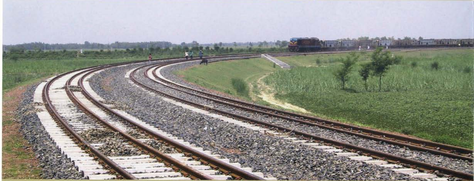
Ishwardi Chord Line and Bypass, Bangladesh
