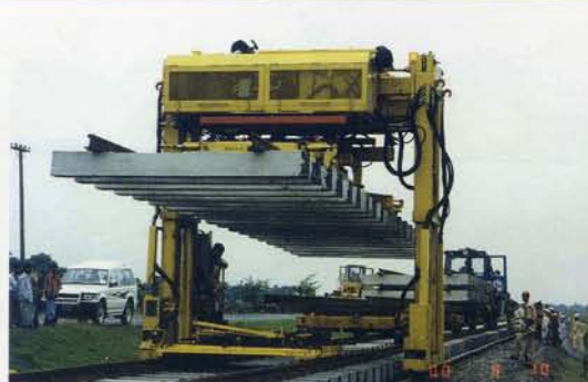
Track lying at Jamuna Rail Link Project, Bangladesh
